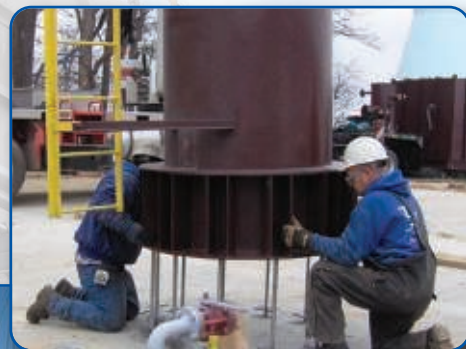
RTO & Stack Installation ▶
