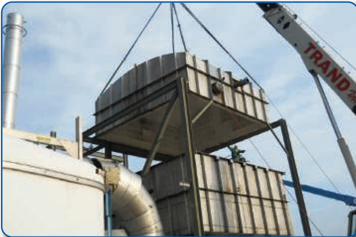
Rotary RTO Rebuild
