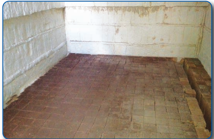
RTO HX Media Replacement & Insulation Hot Spot Repair
