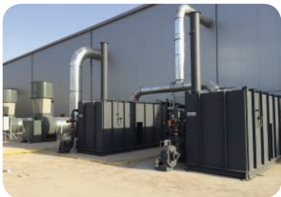
5000 scfm RTO 处理太阳能电池板涂装尾气 5000 scfm RTO for Solar Panel Coating Facility
