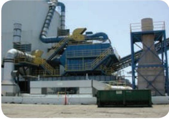
40000 SCFM RTO 处理卤化挥发性有机化合物 40,000 scfm RTO with Acid Gas Scrubber for Halogenated VOCs
